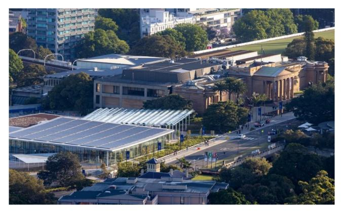
The external facade materials are glass for the public spaces and limestone for the art pavilions, clad in more than 50,000 pieces of hand-cut and hand-laid limestone bricks.
