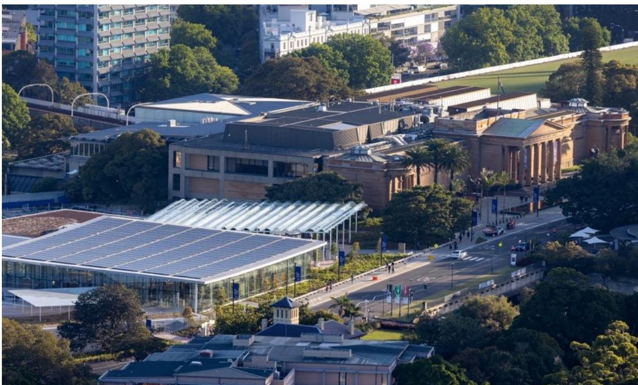
The external facade materials are glass for the public spaces and limestone for the art pavilions, clad in more than 50,000 pieces of hand-cut and hand-laid limestone bricks.
