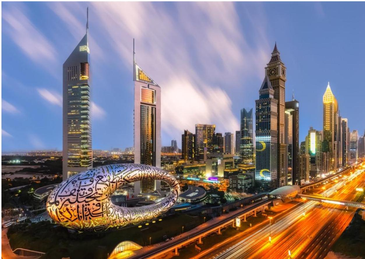
The facade of the building extends over an area of 17,600 square meters. Made of stainless steel, the facade panels were produced using automated robotic arms.
