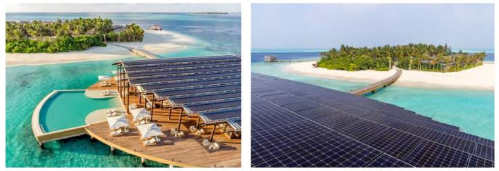
A solar panel system spanning 1643 m<sup>2</sup> – which can be found on the roof of the central hub building known as The Retreat – was designed by Swedish company Solarwork. The full solar installation cost around \$2 million. Total annual production is 575MWh, estimating that Kudadoo will reduce their carbon footprint by 400,000 tons per year.
