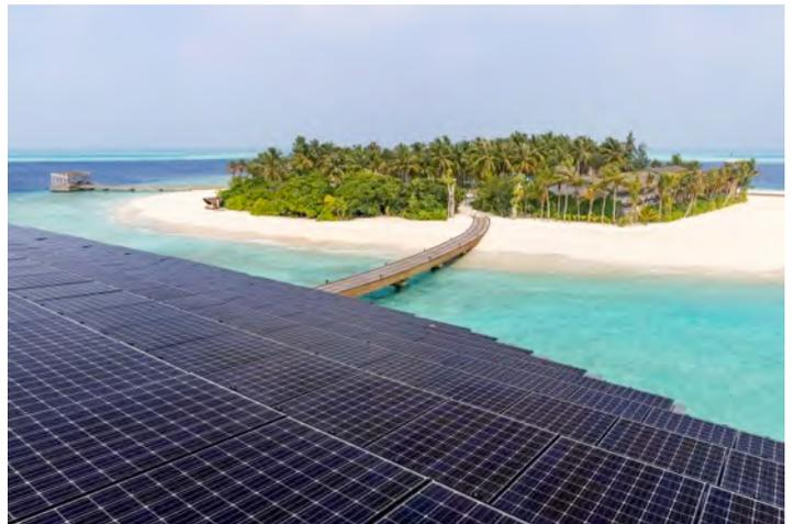
A solar panel system spanning 1643 m<sup>2</sup> – which can be found on the roof of the central hub building known as The Retreat – was designed by Swedish company Solarwork. The full solar installation cost around \$2 million. Total annual production is 575MWh, estimating that Kudadoo will reduce their carbon footprint by 400,000 tons per year.
