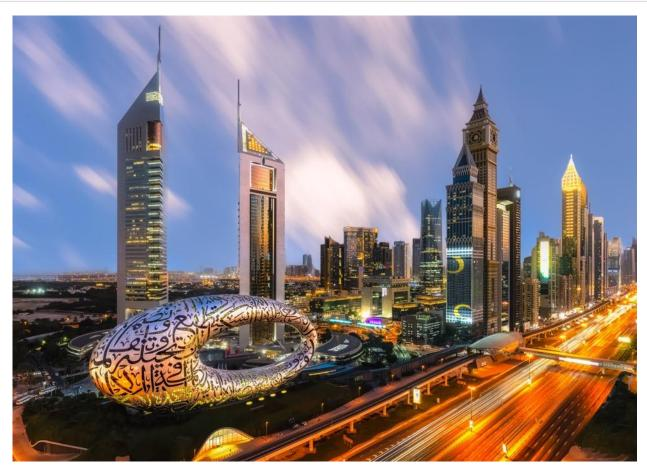
The facade of the building extends over an area of 17,600 square meters. Made of stainless steel, the facade panels were produced using automated robotic arms.
