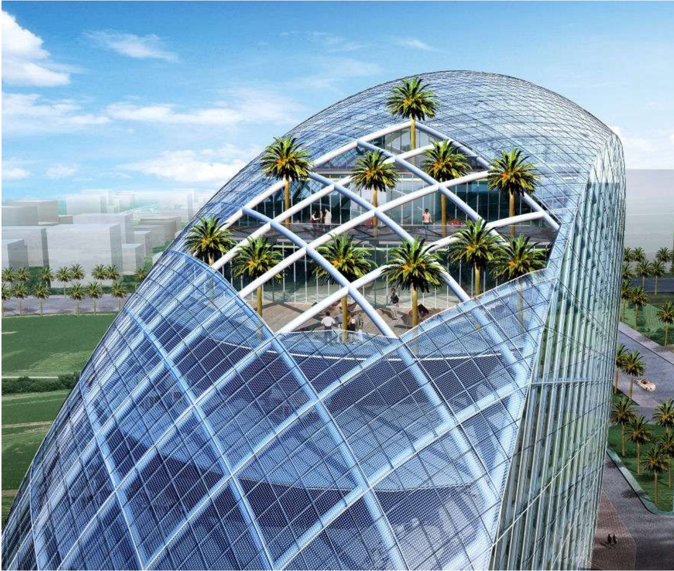
The sky garden on the top of building performs thermolysis (the dissipation of heat from the surface).
