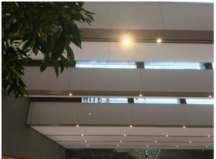
*Raise of the steps are in glass which work as skylight slit on the ceiling from the interior of the store*
